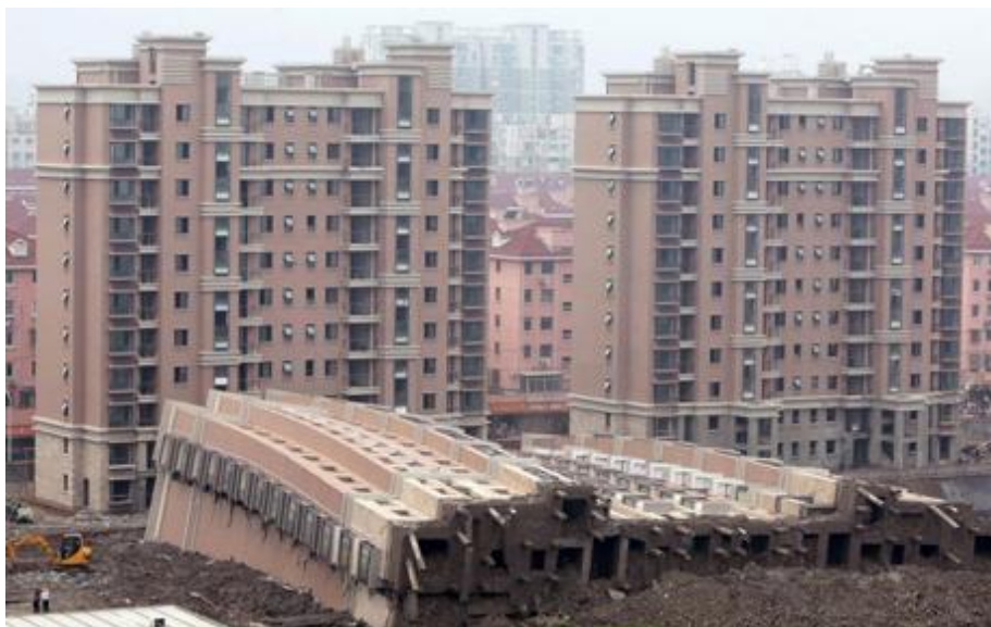
In June 2009, this nearly finished 13-story apartment building in Shanghai just toppled over killing a construction worker. Photo: Reuters
